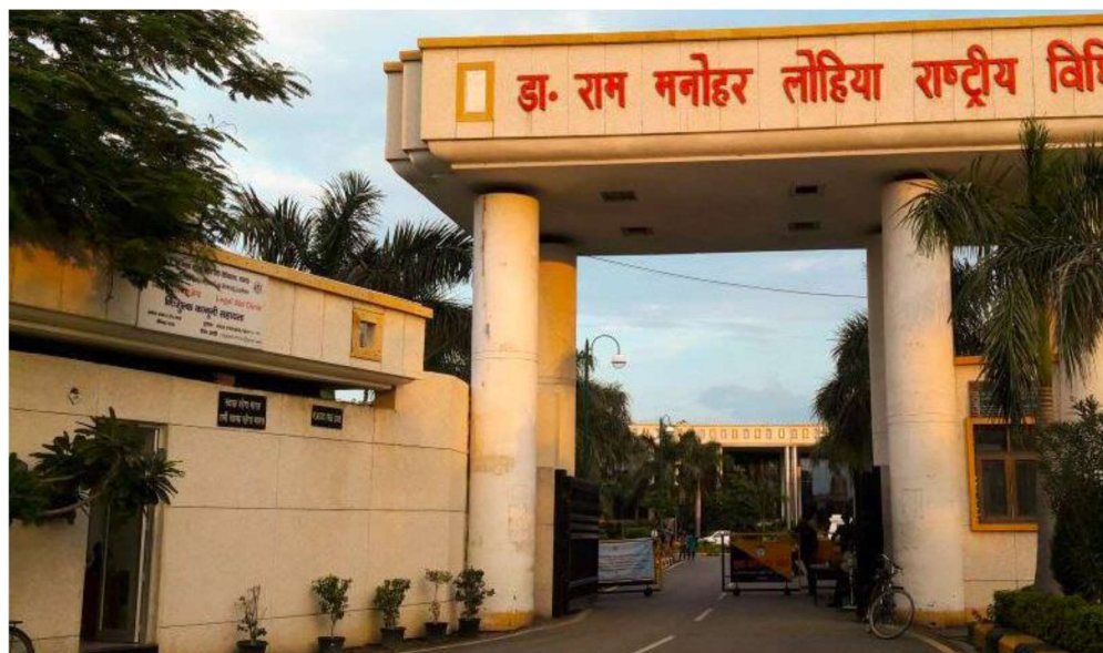
[Legal Aid Clinic on the left side of the main gate of the college]
